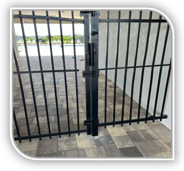
♣ We have been having issues with the gate door closer at amenity 1. The closing device was replaced with a new model which should mitigate further issues.
