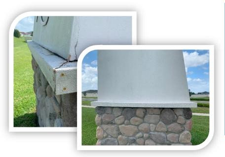
The R monument had weathering and cracking damage. GMS staff cleaned up and repaired the damage.
