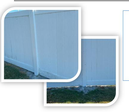
The vinyl fence around the amenity one playground had two posts that were damaged. These have been replaced to help with the fence's structural security.
