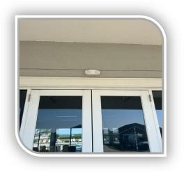
The amenity one emergency light was damaged. It has been replaced with a sturdier light.
