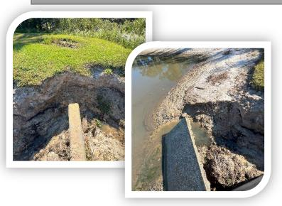
♣ The area south of the weir has eroded from the storm lowering the stormwater pond levels at Salt Springs.
