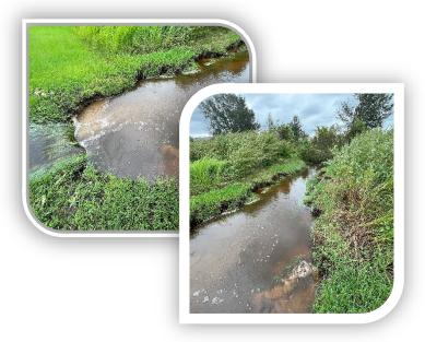
The sump that uses a swale to manage overflow had the swale eroded from the high volume of water.
