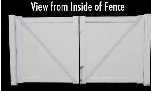
Hinge location dictates gate swing Gate pictured swings out
